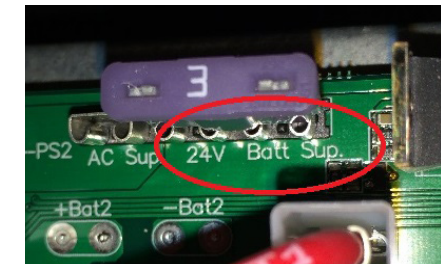
Figure 4: SV control panel power settings
